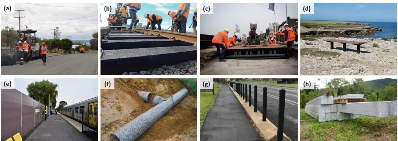
Figure 3.41: Various applications of recycled plastics in road and rail infrastructure: (a) asphalt, (b) railway sleepers, (c) bike paths, (d) plastic furniture, (e) noise wall, (f) pipes, (g) bollards and (h) lumber
