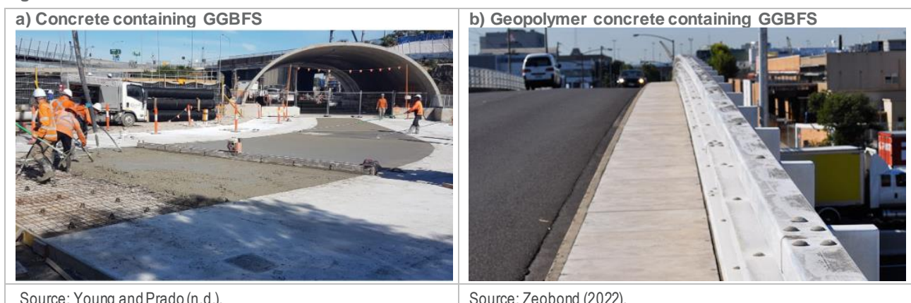
Figure 3.17: Use of GGBFS in concrete works
